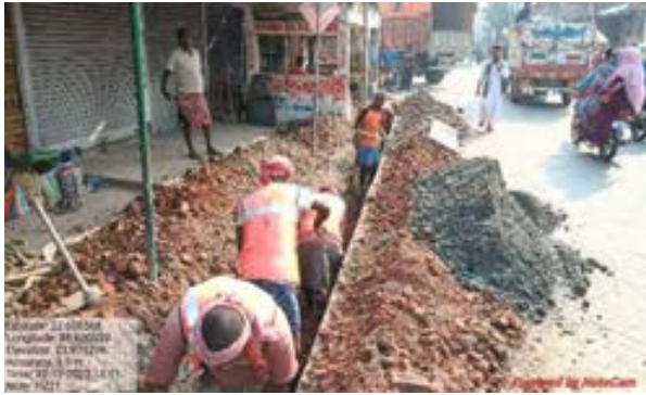
Fig: Zone 21 Pipeline –Partial use of PPEs during pipe laying-Haroa Block
