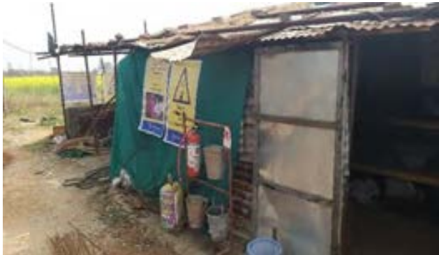
Safety signage, Fire extinguisher noted at Manikmara OHR site
