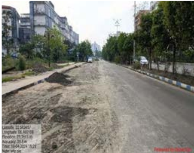
Fig: Partial road restoration in street no- 77- Pipeline work area
