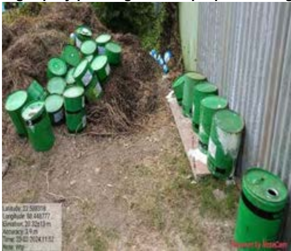
Fig: Empty paint container without platform
