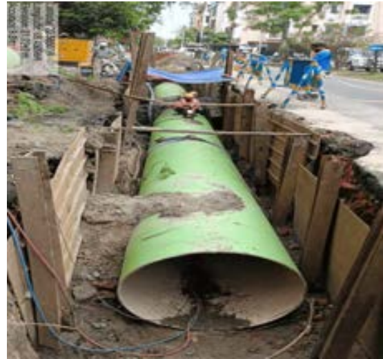
Fig: Satisfactory Use of PPEs at Pipeline laying work area
