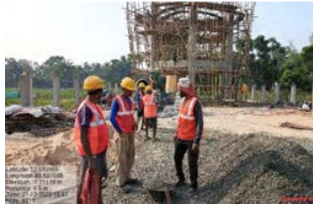
Fig: Zone 11 OHR – Use of PPEs during column concreting-Bhangar-II Block
