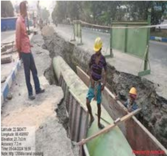
Fig: Partial use of PPEs by workers at Pipeline laying area
