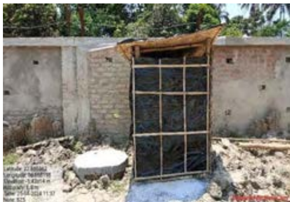
Fig: Provision of twin pit toilet at zone 5 OHR Bhangar-II block
