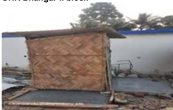
Fig: Completed twin pit toilet at zone 11 OHR Bhangar-II block
