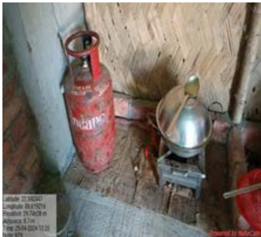
Fig: LPG connection at zone 9-OHR Bhangar-II block
