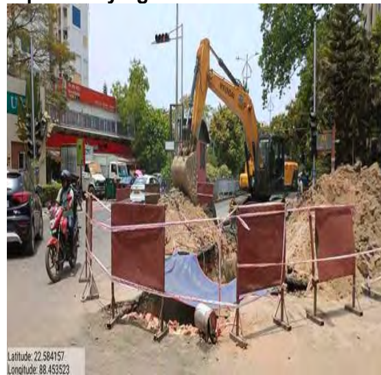
Fig: Satisfactory barricading at pipeline laying area near WTP
