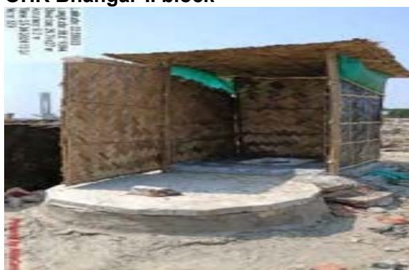
Fig: Twin pit toilet at zone 9 OHR Bhangar-II block
