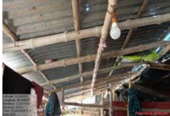
Fig: Zone 5 OHR –Camp shed replaced with metal sheet- Bhangar-II Block
