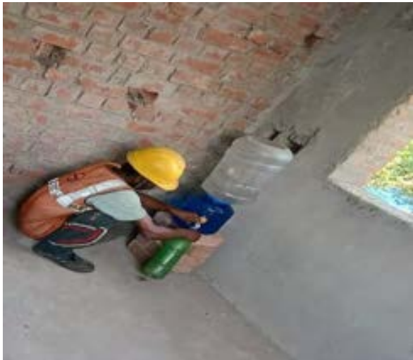
Drinking water arrangement at work site (package BK/04)
