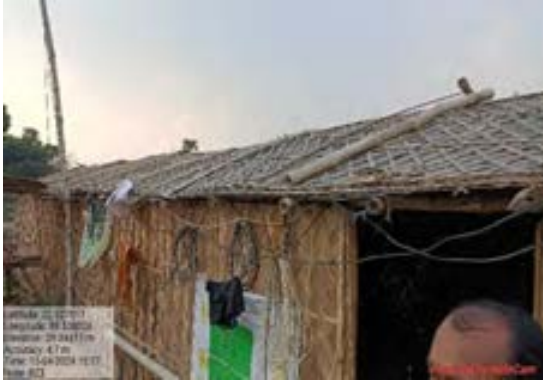
Fig: Zone 3 OHR- Plastic sheet cover in camp at Bhangar-II Block
