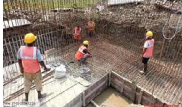
Fig: Zone 3 OHR – Use of PPEs during concreting work-at Bhangar-II Block
