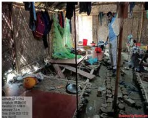
Fig: Damaged camp with bad housekeeping- Bhangar-II GLSR
