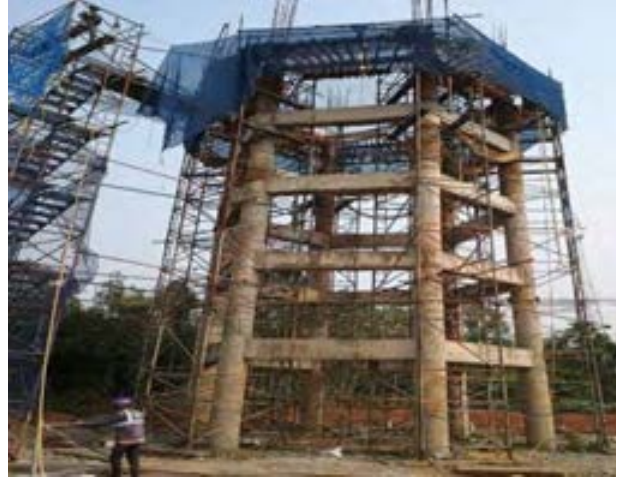
Construction work in progress at BK/02B Fulmati OHR. Safety net noted
