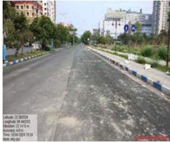
Fig: Full road restoration in street no- 77-Pipeline work area
