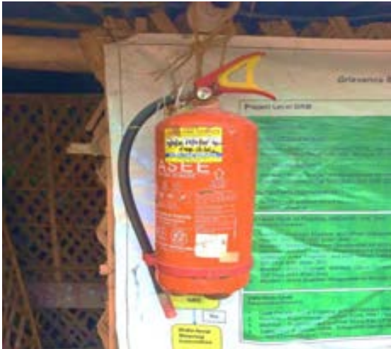
Fig: Filled fire extinguisher in camp area at zone 5 OHR – Bhanagar-II block
