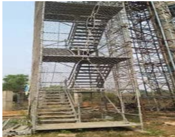
Safety maintained in and around staircase of OHR (package BK/2B)
