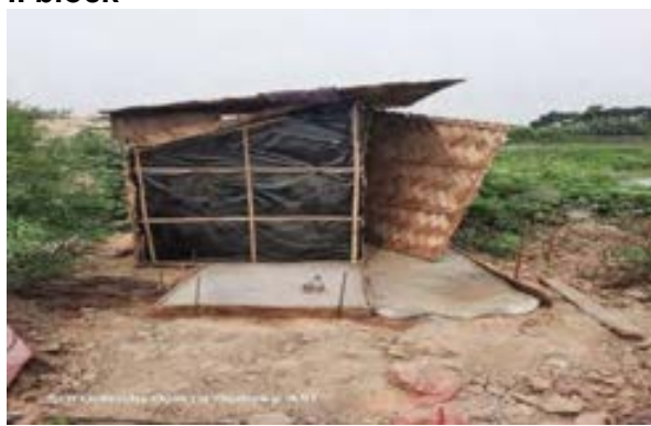
Fig: Replacement by twin pit toilet at zone 14 OHR Bhangar-II block
