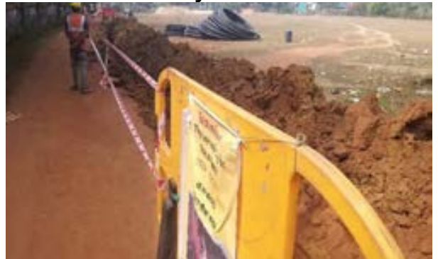
Barricade, caution tape noted at pipelaying location
