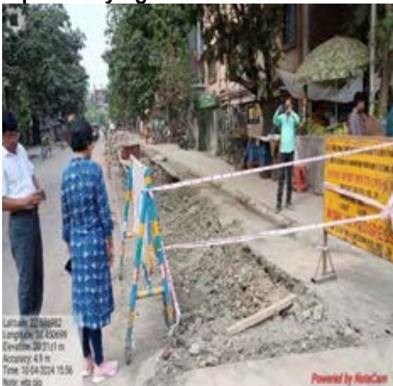
Fig: Partial Barricading at Pipeline laying area near WTP
