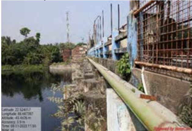
Canal crossing through anchoring at zone 4 OHR -Haroa Block
