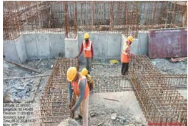
Super Structure Beam construction at CWR-WTP. Use of PPEs noted
