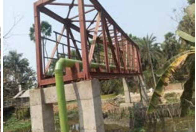
Pipeline and cage work completed at zone-08 canal crossing Bhangar-II Block
