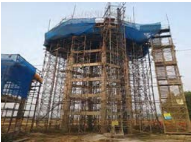
Chakaltore OHR in package Bk/02A under construction. Safety net noted
