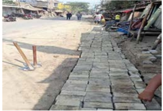
Paved road restoration at zone 21 -PWD road -Haroa Block
