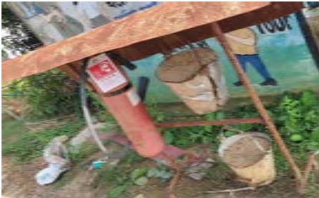
Before: Fire extinguisher near the construction area (Package BK/2B)
