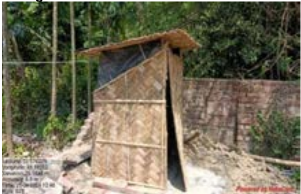
Fig: Newly build twin pit toilet at zone 8 OHR Bhangar-II block
