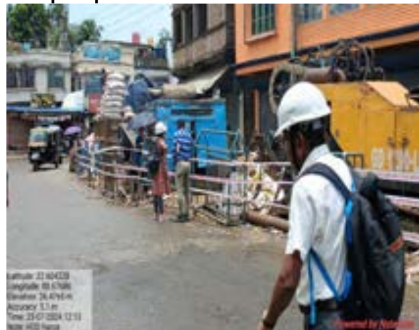
Fig: DSISC team discussed with contractor about improved the barrication & platform.
