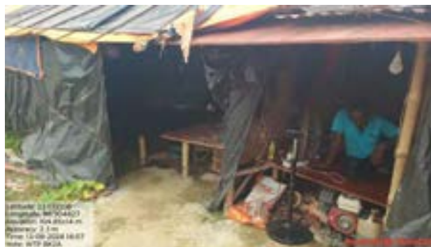
Worker's camp room at Govindapur GLSR site (package BK/01) needs to be improved
