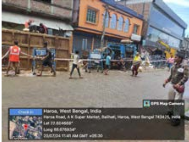
Fig: Satisfactory barricading at working area.
