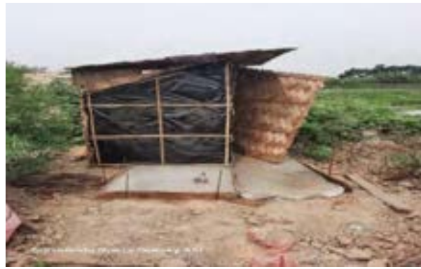
Fig: Replacement by twin pit toilet at zone 14 OHR Bhangar-II block
