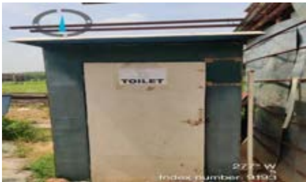
Before: Proper toilet facility was not provided in Package BK/2B
