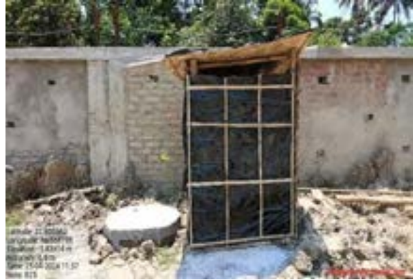
Fig: Provision of twin pit toilet at zone 5 OHR Bhangar-II block
