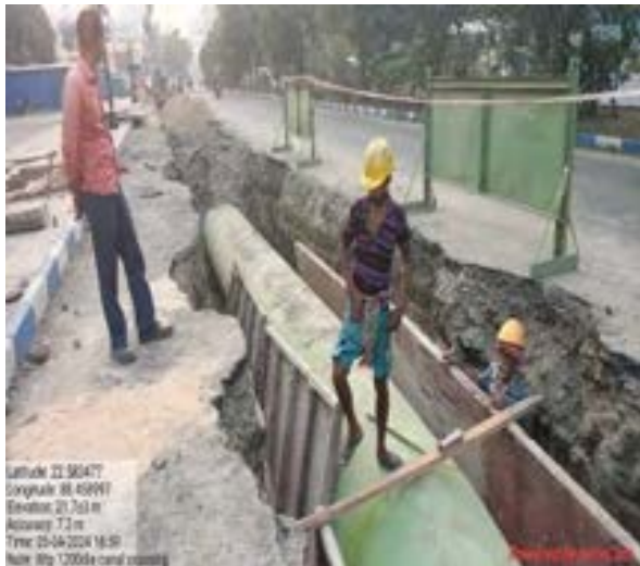
Fig: Partial use of PPEs in Pipeline
