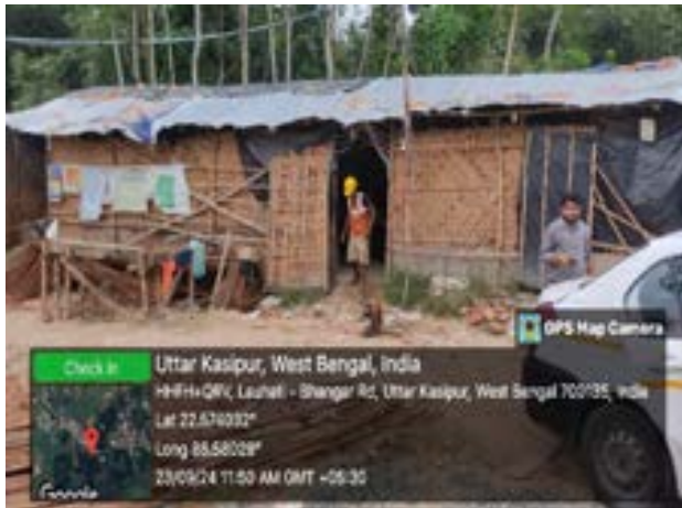
Fig: Zone 8 OHR – Camp shed replaced with metal sheet- Bhargar-II Block
