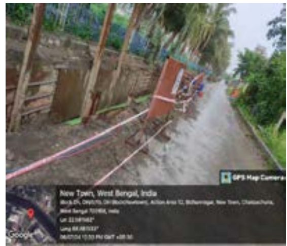
Fig: Satisfactory barricading in pipeline-WTP
