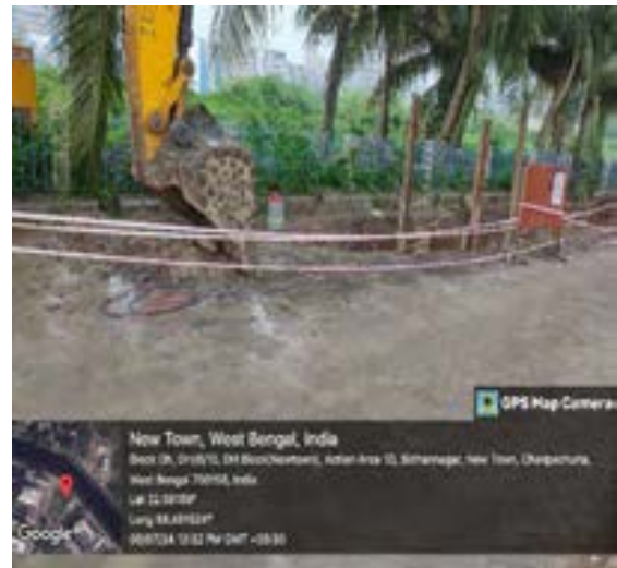
Fig: Satisfactory barricading in pipeline-WTP
