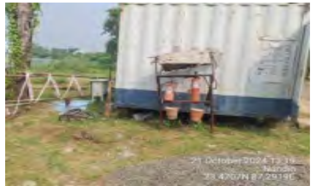
After: Repair of the fire extinguisher shed has been noted
