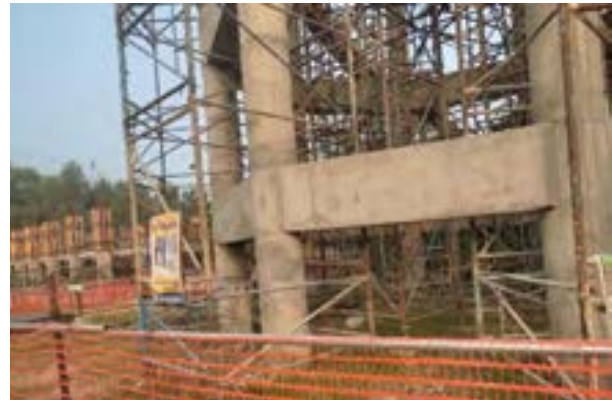
After: Availability of proper housekeeping facility at BK/02A (Govindapur) site
