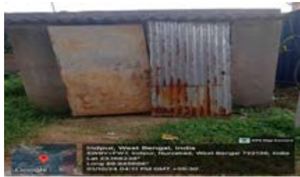
Toilet door has been provided after the instruction (package BK/2A)
