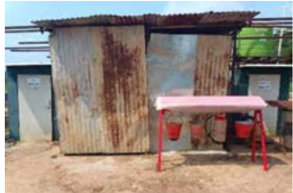
After: New Fire extinguisher installed near the construction area (Package BK/2B)
