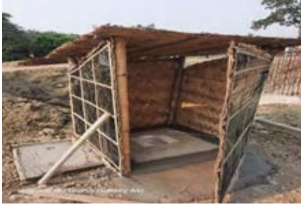
Fig: Twin pit toilet constructed at zone 3 OHR Bhangar-II block
