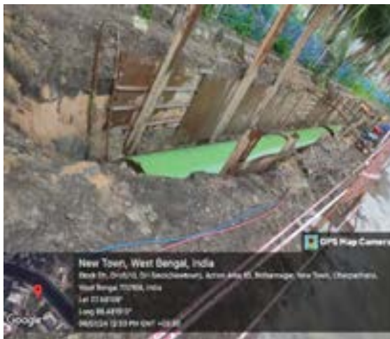
Fig: Satisfactory barricading in pipeline-WTP
