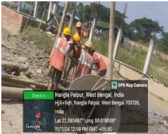
Fig: Zone 9 OHR – Working with PPEs in piling work-Bhangar-II Block
