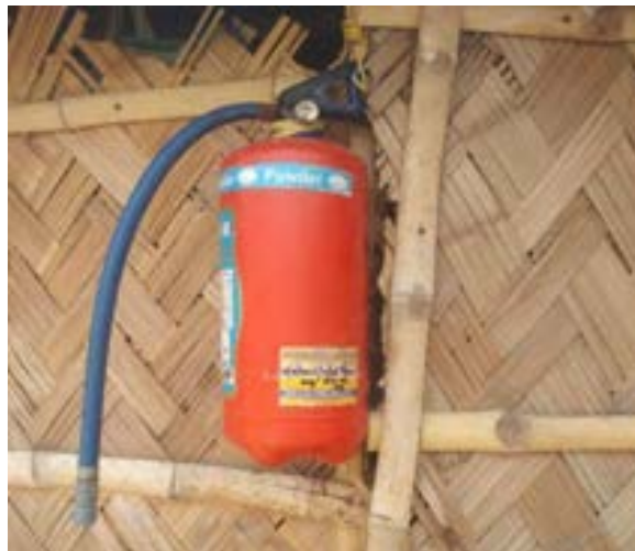
Fig: Replaced fire exitungusher at zone 9 –OHR Bhangar-II block
