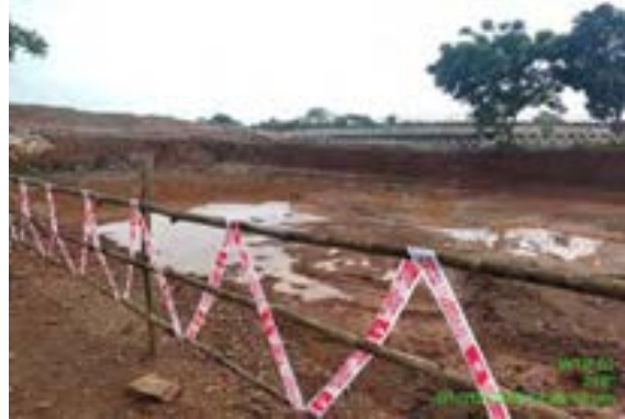
After: Immediate barricading done after necessary instruction
