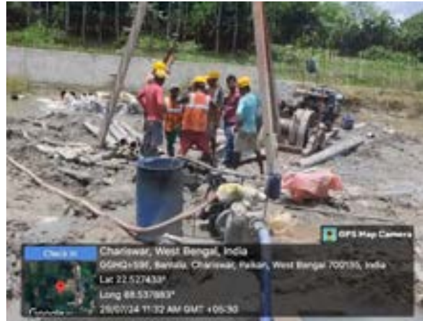
Fig:, Zone 3 OHR – Working with PPEs in piling work-Bhangar-II Block
