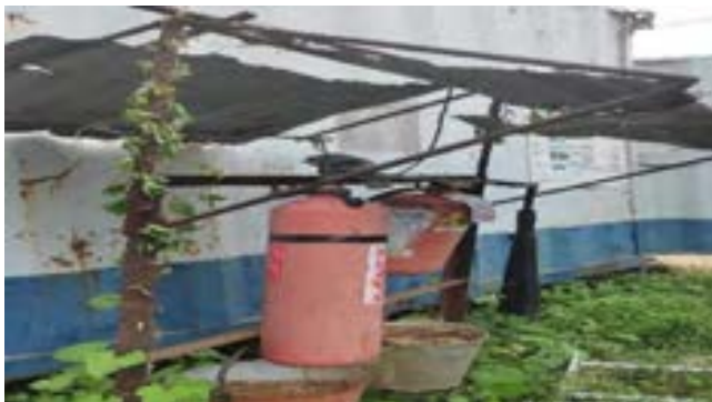
Before: Fire extinguisher near the construction area (Package BK/03)
