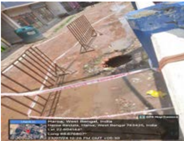
Fig: Satisfactory barricades around the area where the holes were made
