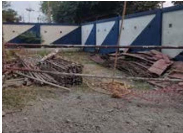
Proper housekeeping at OHSR site (Bk/04)
