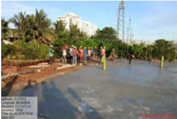
Casting Work at CWR of Bhangar GLSR
