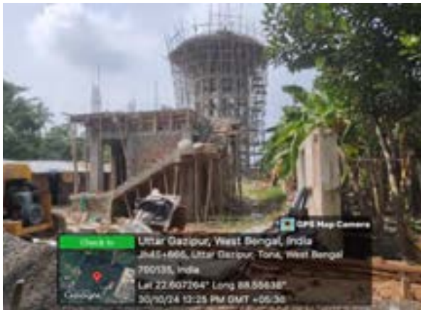
Superstructure work is in progress at Zone -5, Bhangar II block
