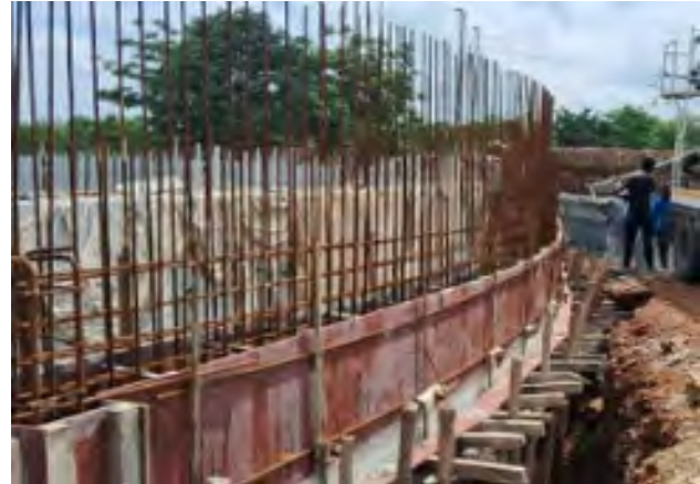
Construction activities at WTP(Bk/01)
