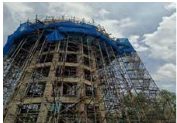
Use of safety net during height work (Bk/02B)
