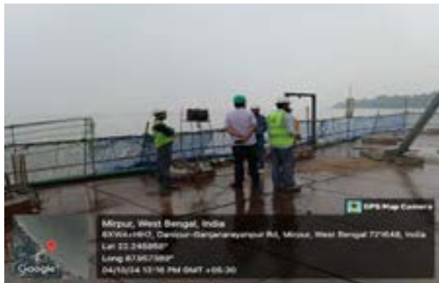
Environmental safety measures at Intake (EM 01)
