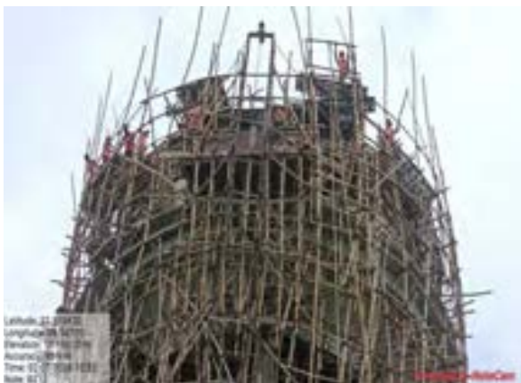
OHR construction work is in progress at zone 11, Bhangar II
