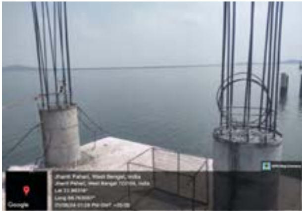
Piling work continued at Intake site (Bk/01)
