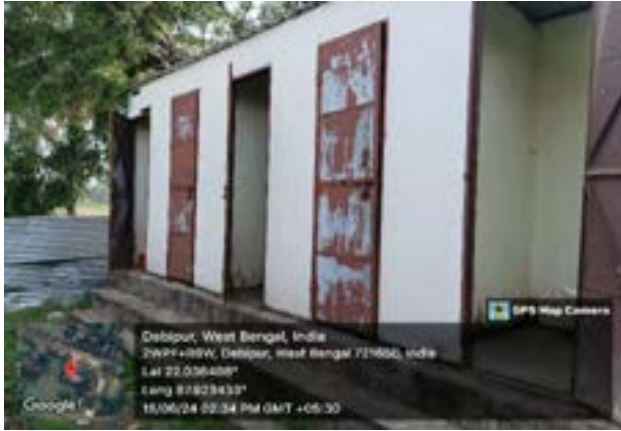
Toilets and washroom available for the workers at Thakurchak Labour colony (EM/02)
