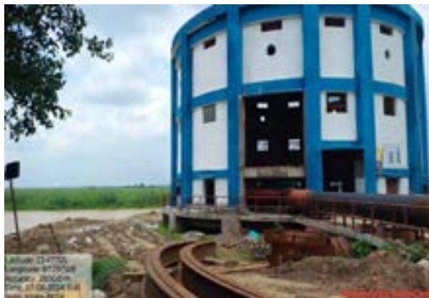
Construction activities at Intake area (Bk/03)
