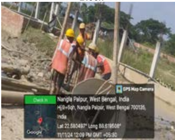
Fig: Zone 9 OHSR – Working with PPEs in piling work-Bhangar-II Block
