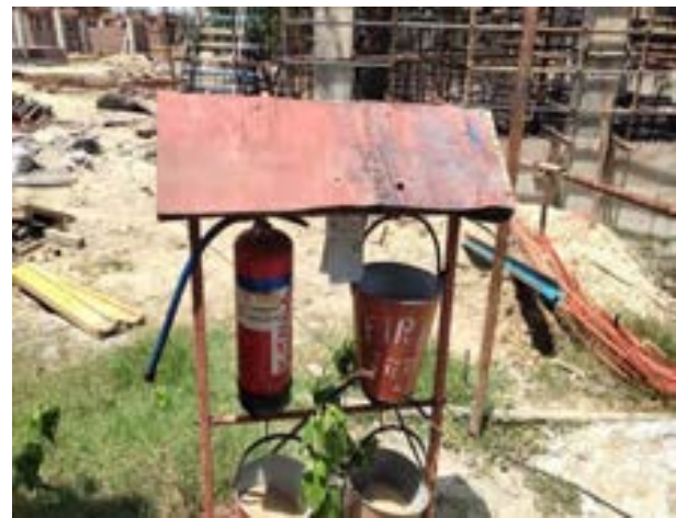
After- They have provide shade to the fire extinguisher. (Package BK/02A)
