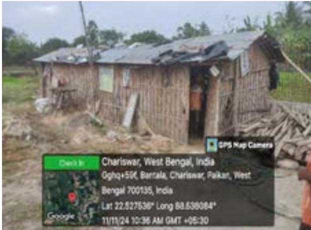
Fig: Zone 3 OHR- Camp shed replaced with metal sheet- Bhangar-II Block
