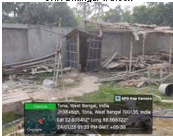
Fig: Twin pit toilet at zone 5 OHR Bhangar-II block
