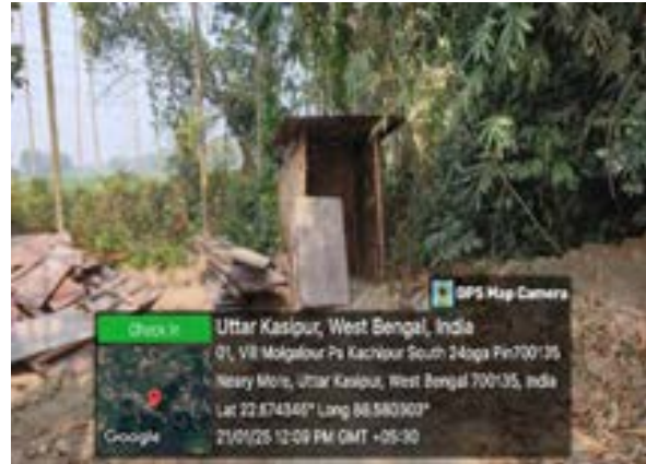
Fig: Twin pit toilet at zone 8 OHR Bhangar-II block
