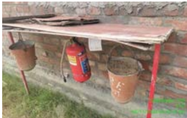
After: Repair of the fire extinguisher shed has been noted
