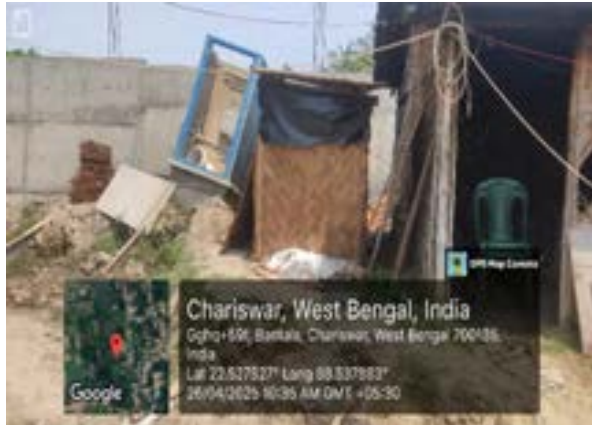
Fig: Newly build twin pit toilet at zone 3 OHR Bhangar-II block
