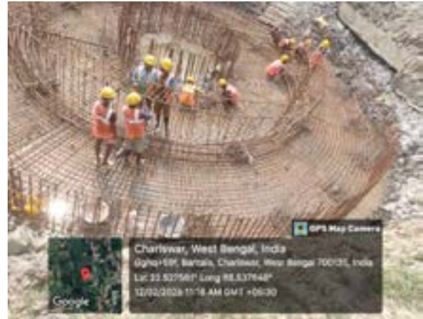
Fig:, Zone 3 OHR – Working with PPEs in OHSR foundation work-Bhangar-II Block
