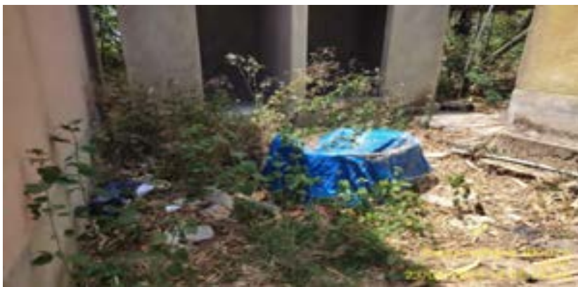
Worker's toilet access needs to be cleaned
