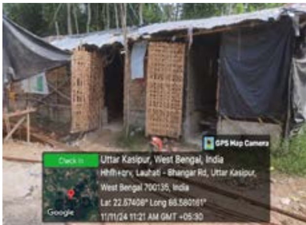
Fig: Zone 8 OHR – Camp shed replaced with metal sheet- Bhangar-II Block
