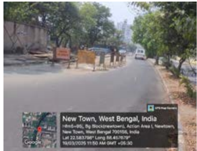
Fig: Barricading during Pipe laying near Canal Location, New Town
