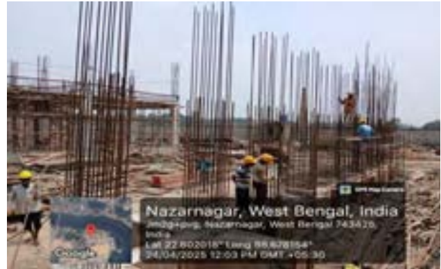
Haroa GLSR Substation outside column reinforcement work on going. (PACK N24PGS/01)
