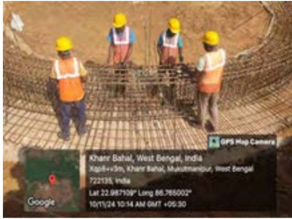
Construction activities at WTP (Pack BK/01)
