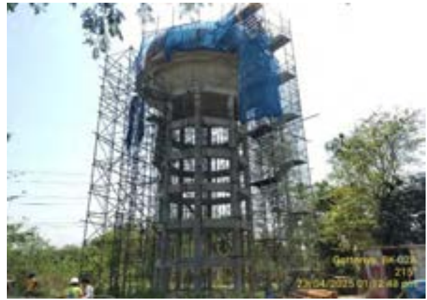
Civil work continued for Pack Bk/02A
