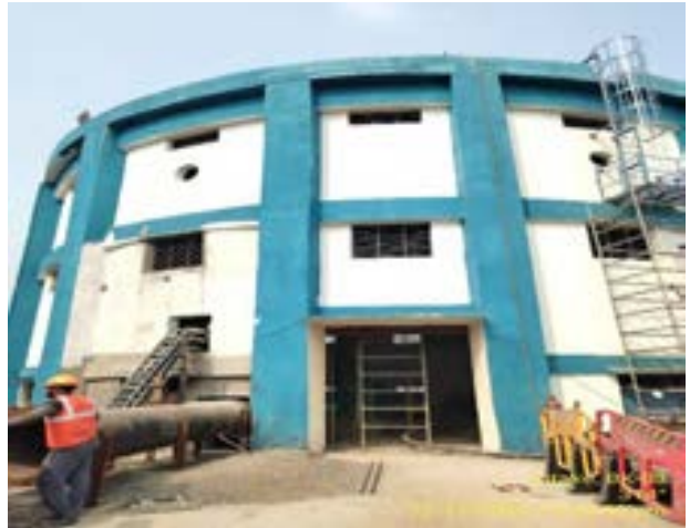
Construction of intake completed Pack Bk/03
