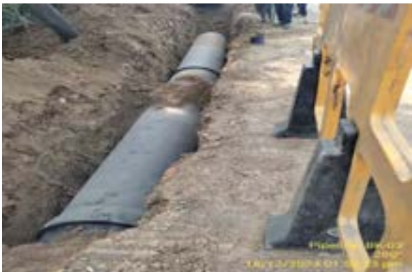
Safety during working at pipelaying site Pack Bk/03
