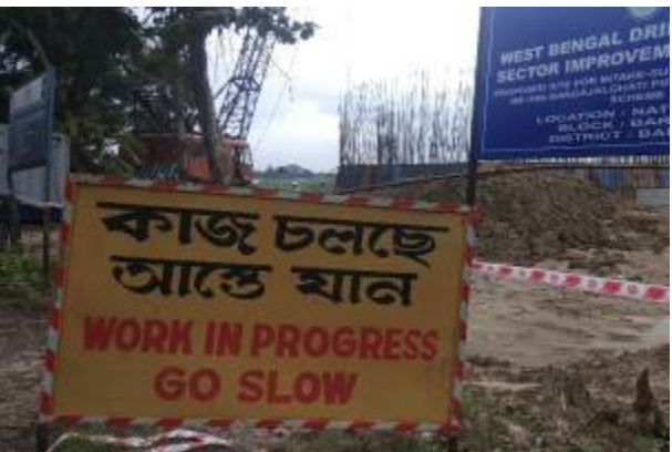
Safety sigange near intake point construction site
