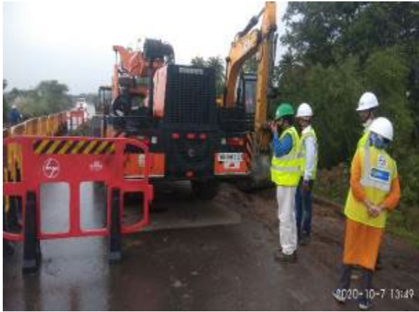
Pipe laying activity for transmission main. Barricading noted
