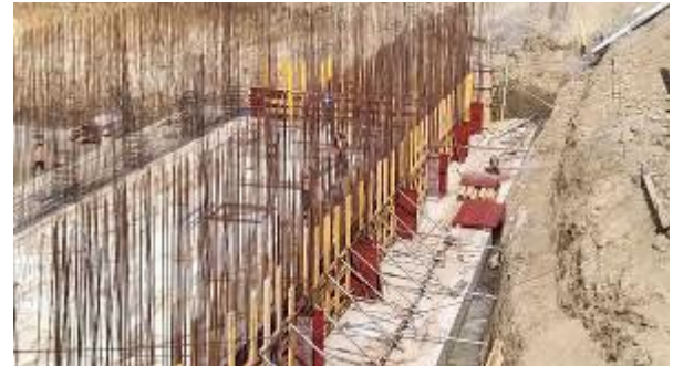
Construction ongoing for WTP
