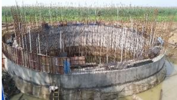
Construction of intake within Durgapur barrage under package BK/03 continued
