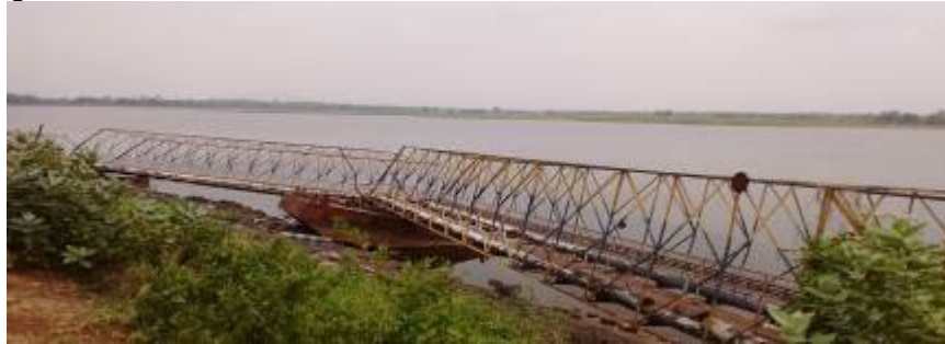
Sali reservoir and the raw water main
