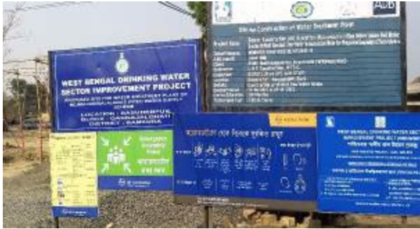
Project display board, emergency contact no board and GR board available at entry point of WTP under Pack BK/03
