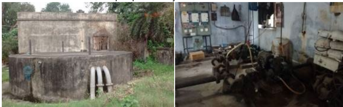
Existing ground level reservoir and pump house
