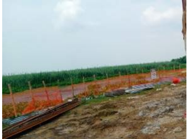
Barricading at intake site under construction
