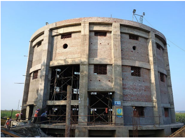
Construction ongoing on at Intake Point
