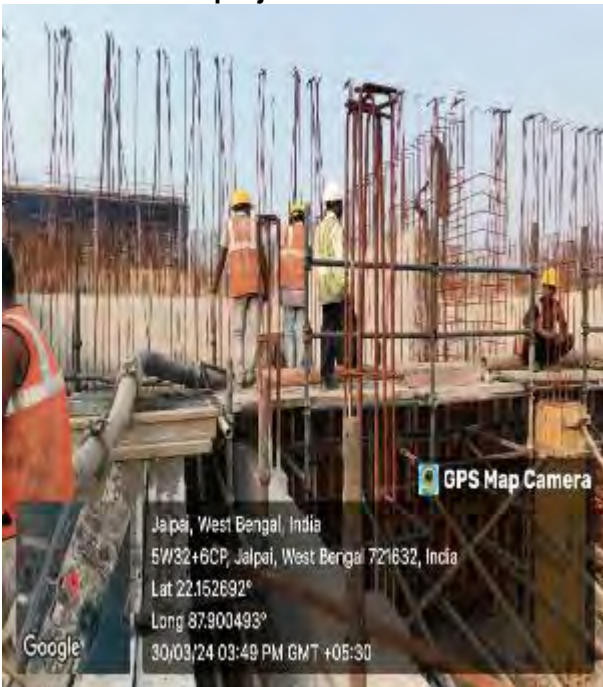
RC wall concreting work at WTP
