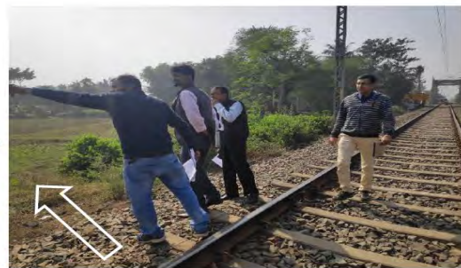
From here it will cross the rail way crossing through trenchless method
