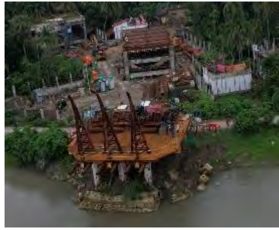
Sub-station and pump house location
