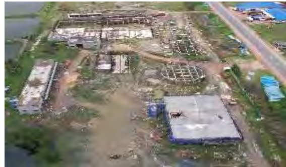
WTP site- work continued
