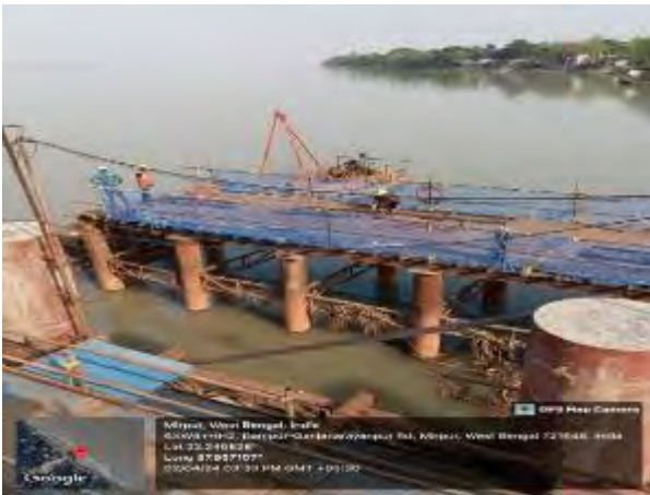
Boring work at Intake Approach Bridge
