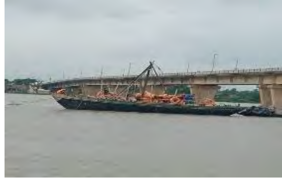
Narghat bridge crossing - Soil testing continued
