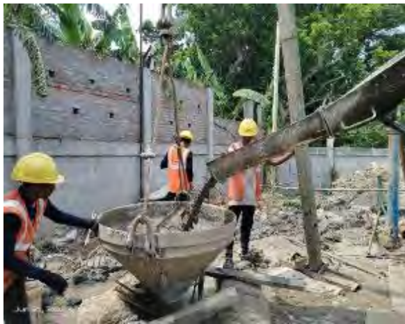
Pile concreting in Admin cum SCADA building at Intake site
