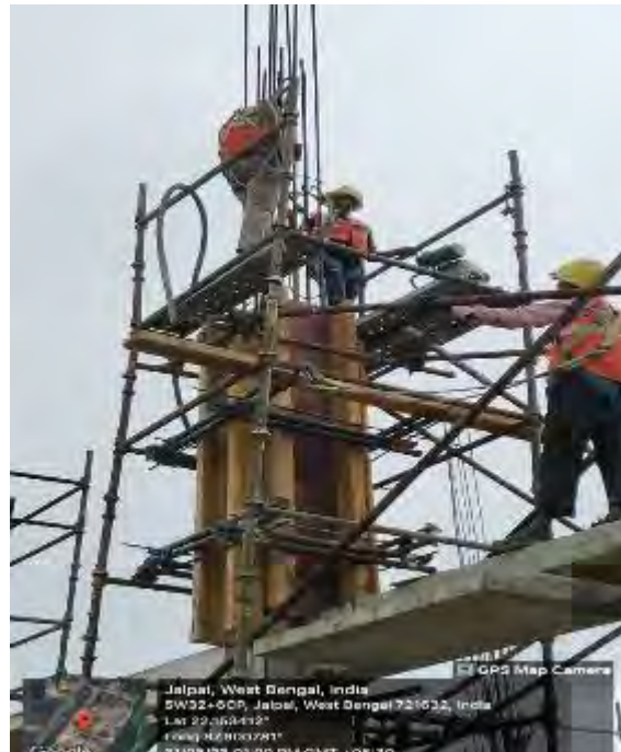
Column casting of Chemical house at WTP
