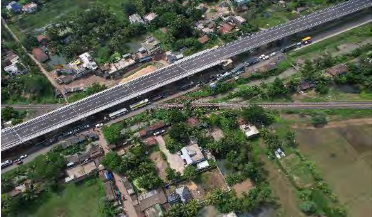
Magrajpur Railway crossing
