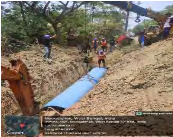
CWRM Pipe laying work in progress near Mangalchak
