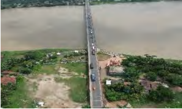
Haldi River - Narghat bridge crossing - Pipe crossing bridge will be constructed
