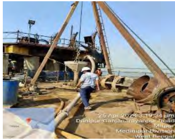
Piling works in progress at Intake Pump house
