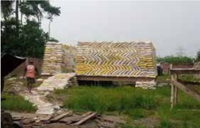
Load test for column at zone -5 OHR, Bhangar-II Block
