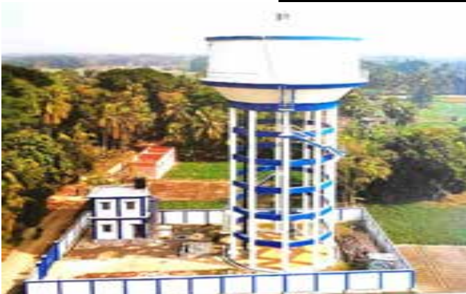
Superstructure at zone-16 OHR, Bhangar-II Block completed
