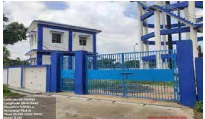
Superstructure at zone -12 OHR, Bhangar-II Block completed
