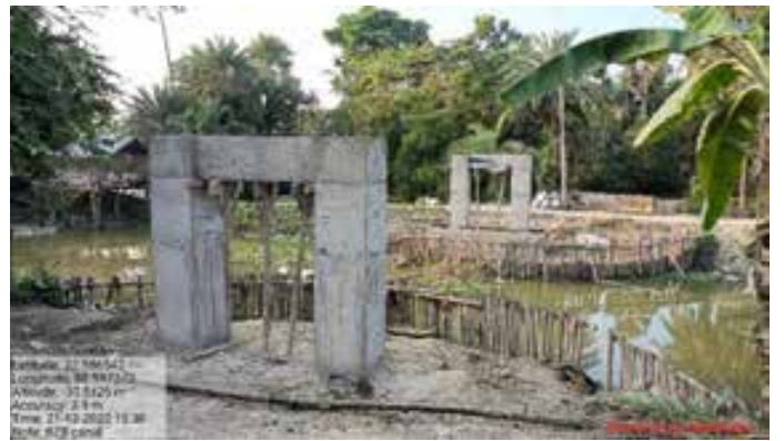
Cage structure at zone -8 Pipeline crossing, Bhangar-II Block
