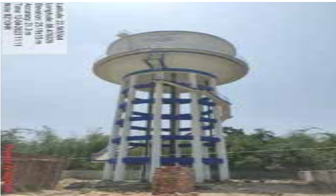
Superstructure at zone -6 OHR, Bhangar-II Block
