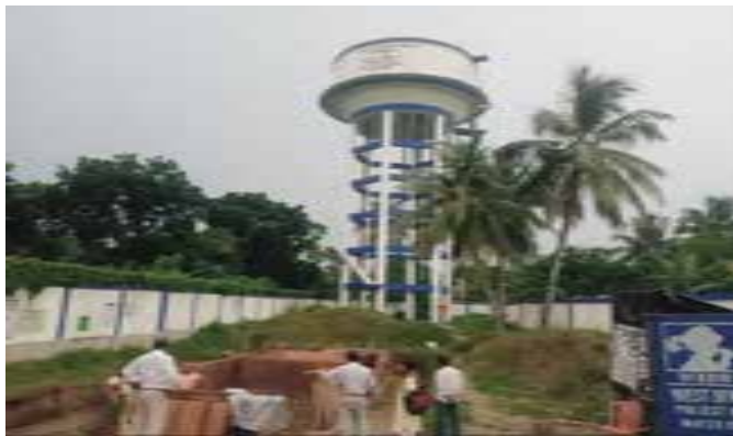
SCADA building work at zone -6 OHR, Bhangar-II Block
