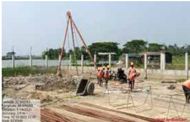
Piling work at zone -9 OHR, Bhangar-II Block
