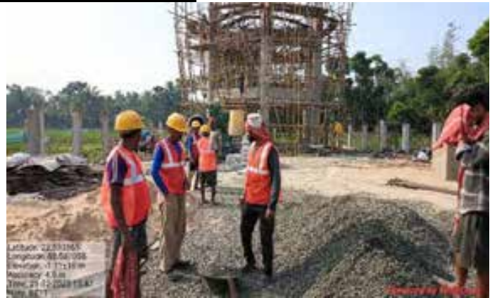
Column Concreting at zone -11 OHR, Bhangar-II Block
