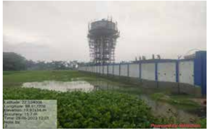
Completed superstructure at zone -2 OHR, Bhangar-II Block
