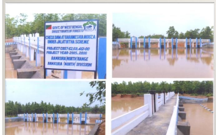
Figure 45: Check Dam in Bankura
