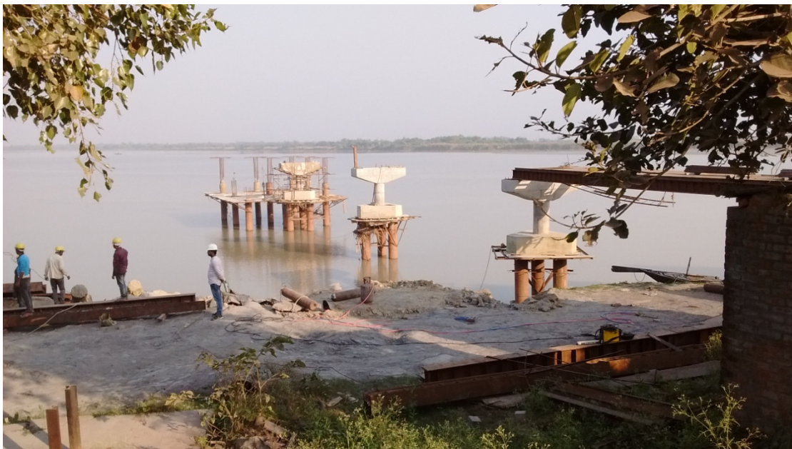
Figure 15: Intake on the river Rupnarayan
